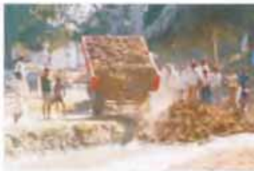
Earth Work through Shramdams
